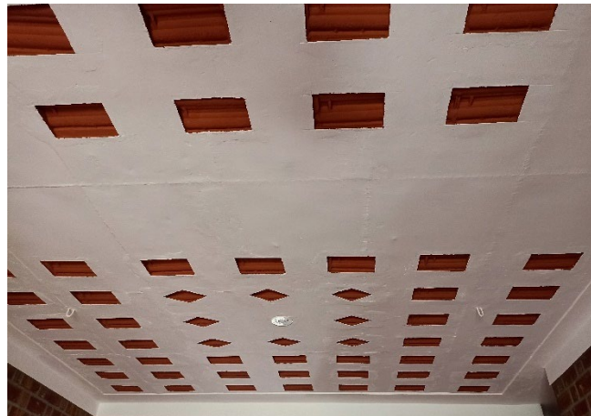
Fig: Final finishing of Filler slab
