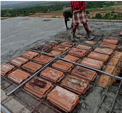
Fig: Filler slab Casting with MP tiles as Filler
