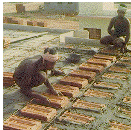
Filler slab Roofing
