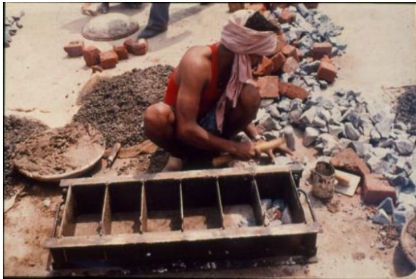
Fig: Fill the stones 50-70 mm in size. Fill in lean concrete in between the stones and compact with plate vibrator
