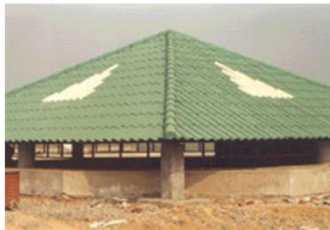
MCR Tile roofing
