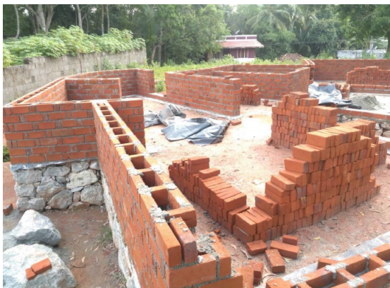
Fig: During Construction
