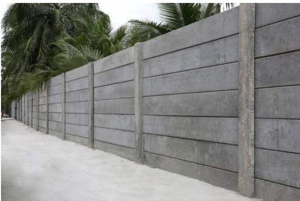
Fig: Precast concrete panels fixed to the concrete pillars
