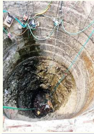
A well being filled by the water supplied from a well in a nearby village via pump. However, people have connected their own motor pumps in the main pipe to take water into their homes thus leaving very less water in the well
