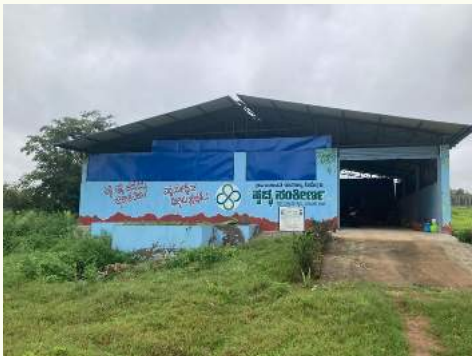
Solid Waste Management Shed
