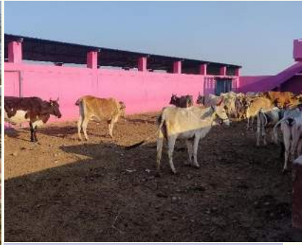
Cow Shelter (Gaushala) made under MGNREGA
